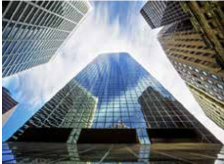
Safety equipment in buildings opened to the public
